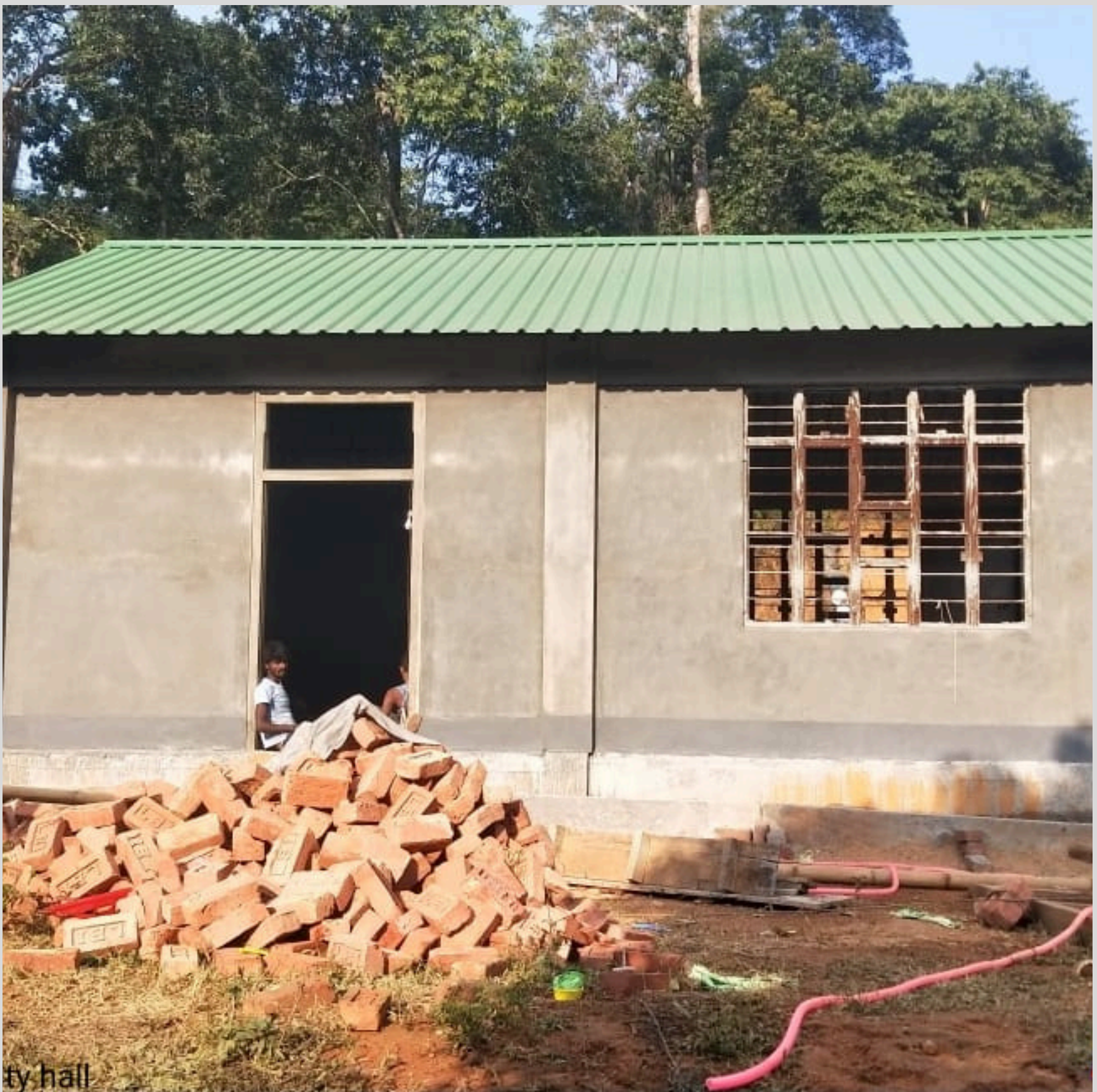
3rd Phase progress of Community Hall, in Bangsi Minol VPIC
